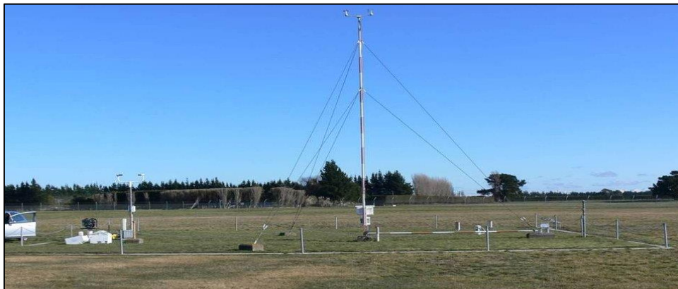
Automated Ceilometer Station for the 2 main meteorological airport offices
